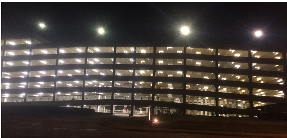
Retrofitted garage on left. Previous lighting system on right
